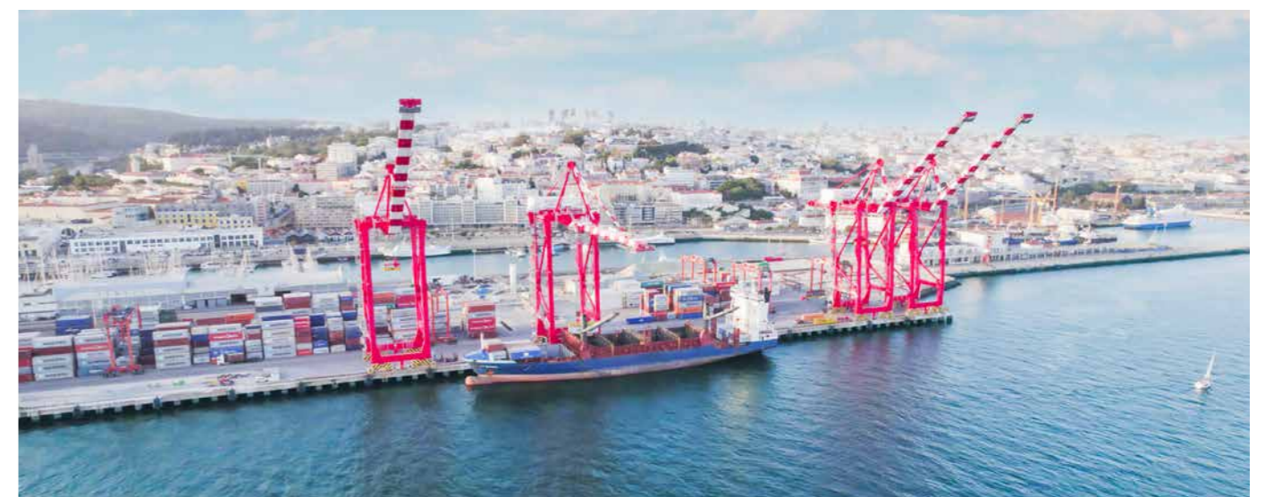
Below First Operations with New STS Cranes
