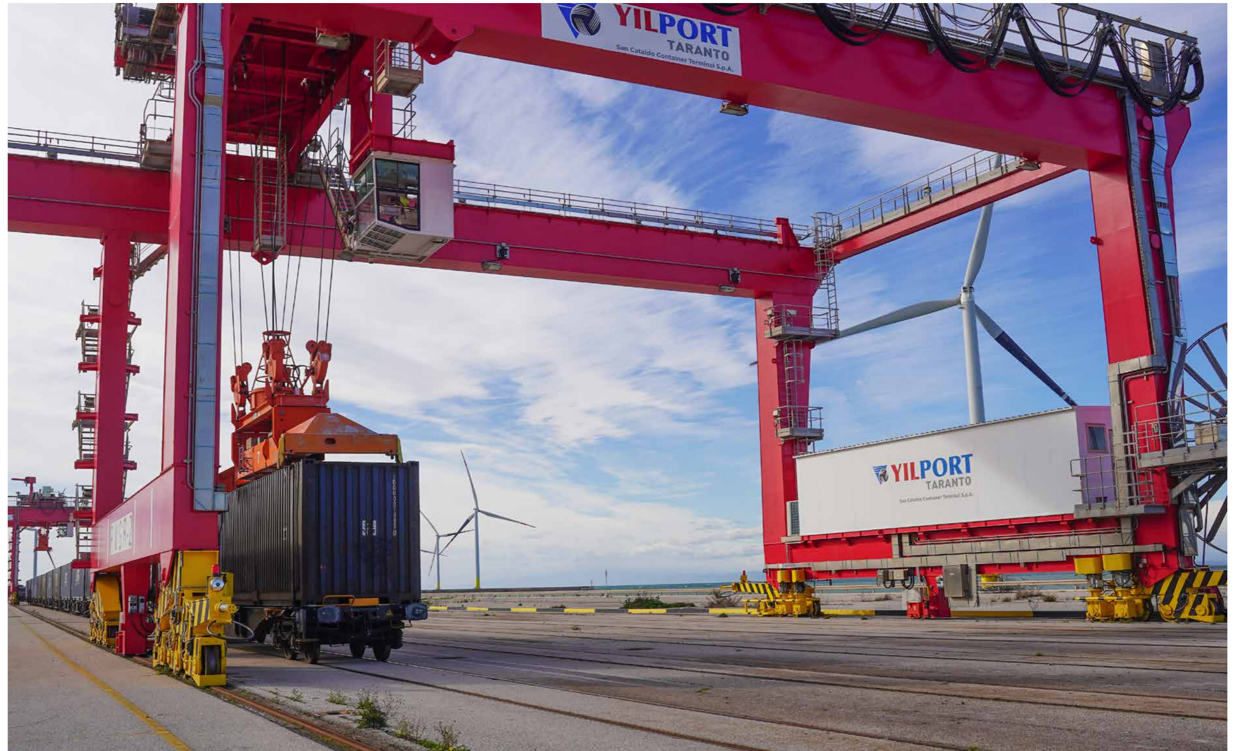
Above YILPORT Taranto San Cataldo Container Terminal
