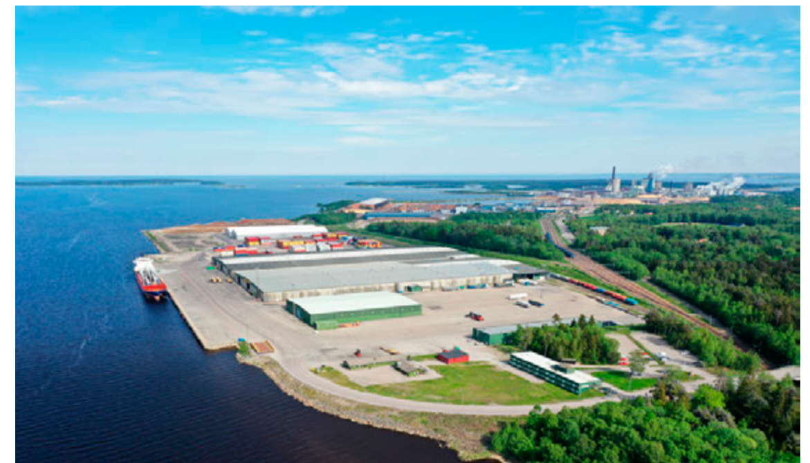
YILPORT Gävle General Cargo Terminal, Sweden
