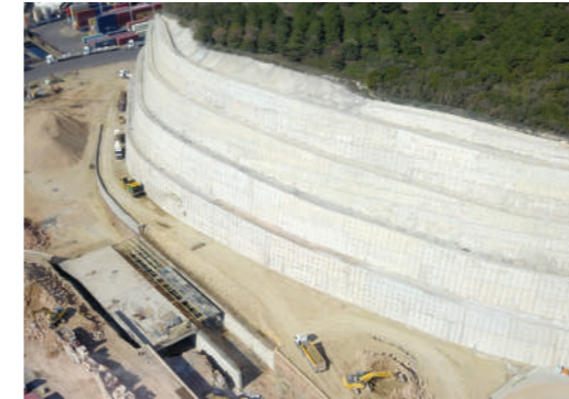
Earthwork and Retaining Wall Construction
